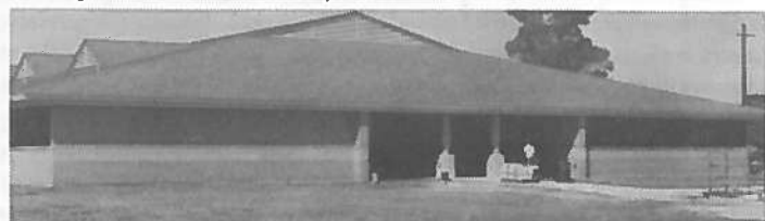
NEW CENTER —A new $3 million Aquaculture Research/Extension Facility soon will be ready at the Agricultural Center's Ben Hur Farm research unit south of the campus.
